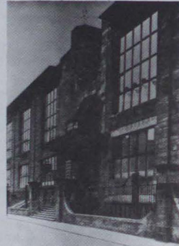
North Facade, Glasgow School of Art, 1899-1907
