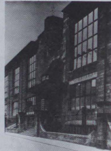
North Facade, Glasgow School of Art, 1899-1907
