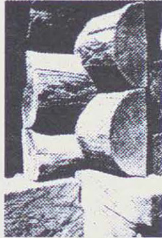
Log construction corner joint in Kosiw, Carpathian Region. Photo: P.H. Yurchenko
