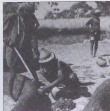
A Batammaliba earth-priest folds the ritual bundle, the tatati , into the building's foundation. Both the intangible symbolic action of the ritual and the tangible symbolic object, the tatati , will remain a part of the completed building. (Blier, 25.)
