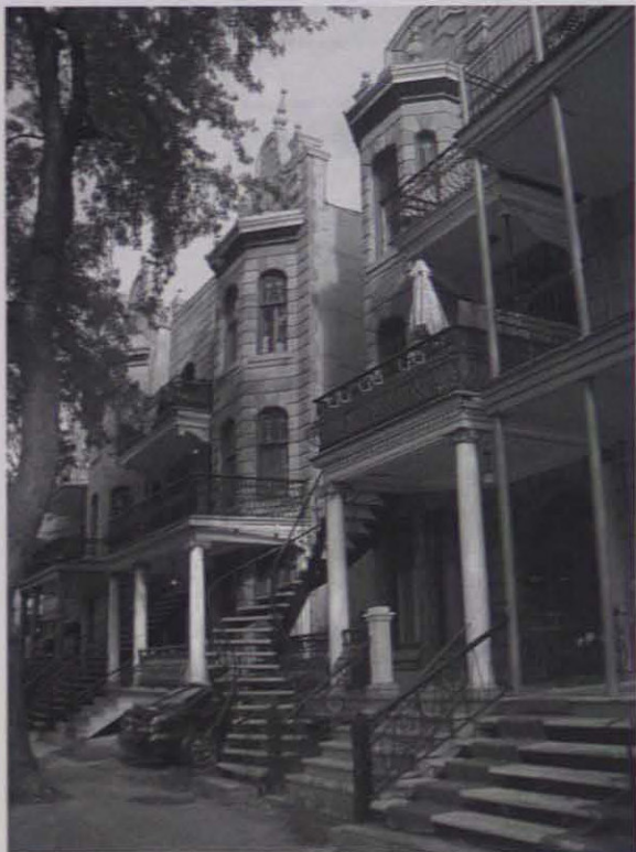
Figure 6. Serpentine staircase, rue Saint-Hubert.
