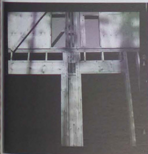
wood framing connection
